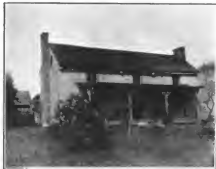
THE E. M. BRANK HOUSE, GREENVILLE
